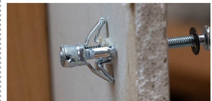
Step 5: Unscrew the screw, put it in a hanger.
